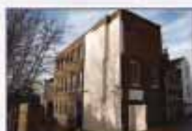
MARGATE Large Commercial Premises Guide: £130-150,000
